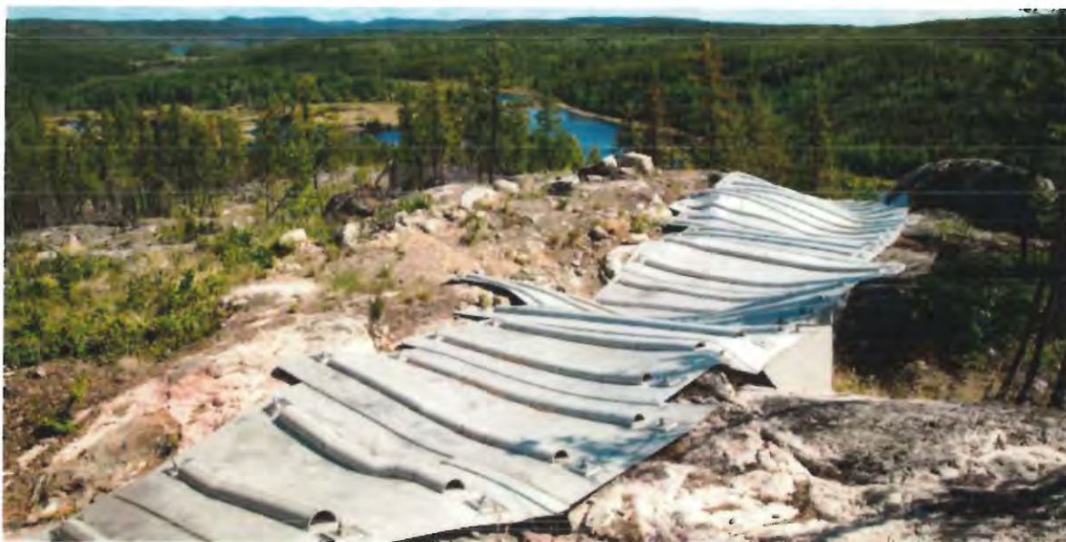
Figure 6: Pre-fabricated Stainless-steel Stope Closure at Rix-Athabasca, Leonard Mine, Saskatchewan
